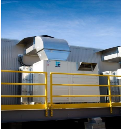
Ducted System – high end solution typically used in extreme hot/cold environments & industry specific
