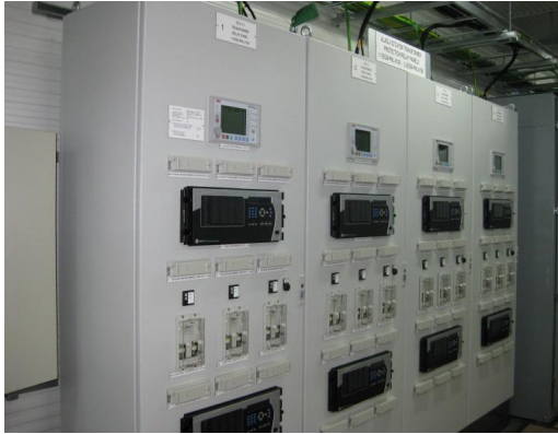
Relay Protection, Generator Control Panels & Misc Control Panels
