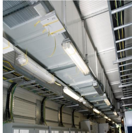
Ducted System – high end solution typically used in extreme hot/cold environments & industry specific
