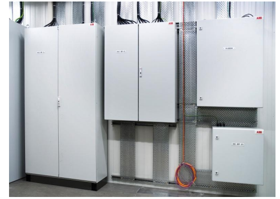
Relay Protection, Generator Control Panels & Misc Control Panels
