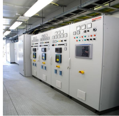
Relay Protection, Generator Control Panels & Misc Control Panels
