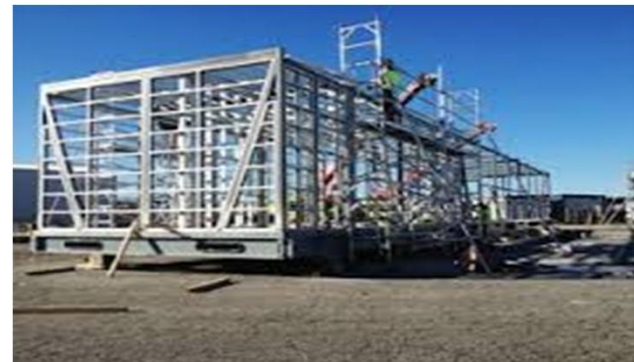
Walls & Roof Frame – fully welded or bolted sections.
