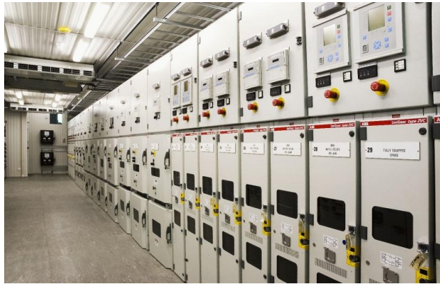
IEC or ANSI Medium Voltage GIS & AIS Switchgear (3.3kV to 33kV)
