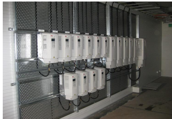
Variable Speed Drives can be wall mounted as option to being inside MCC's
