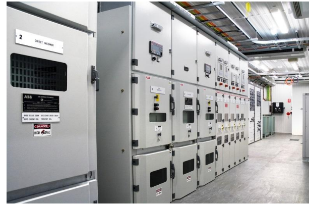
IEC or ANSI Medium Voltage GIS & AIS Switchgear (3.3kV to 33kV)
