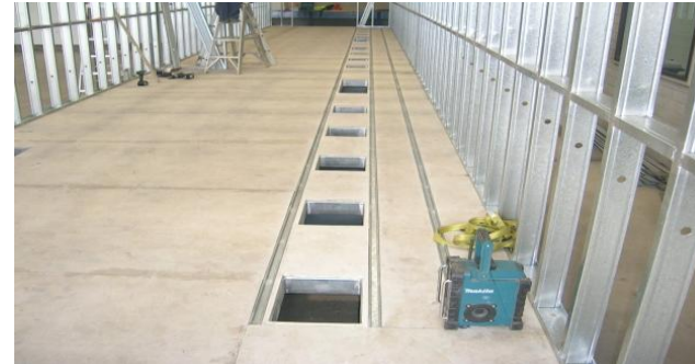
Base Frame – fully welded, custom designed to suit equipment loadings and cable penetrations
