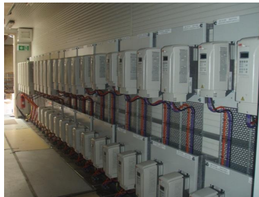
Variable Speed Drives can be wall mounted as option to being inside MCC's
