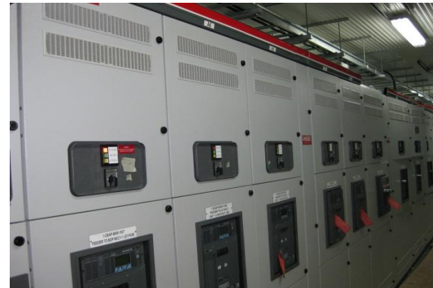
IEC or ANSI Low Voltage Switchgear & MCC's (380V – 690V)
